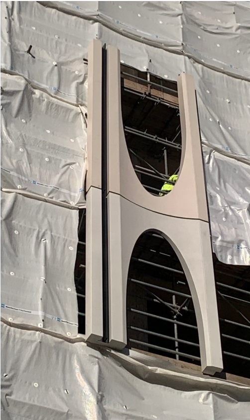
On-site mock-up of elliptical module
