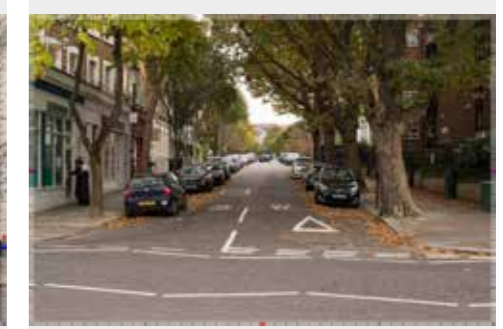
11 | Outside Toilets At westbourne Grove And Denbigh Road
