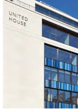
United House, Notting Hill Gate
