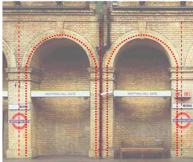
Arched openings to Notting Hill Gate Tube Station
