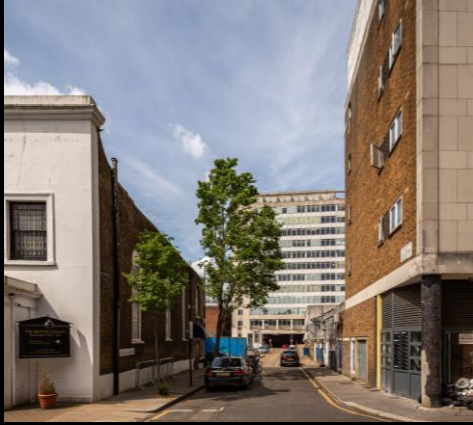
Existing Site Condition
