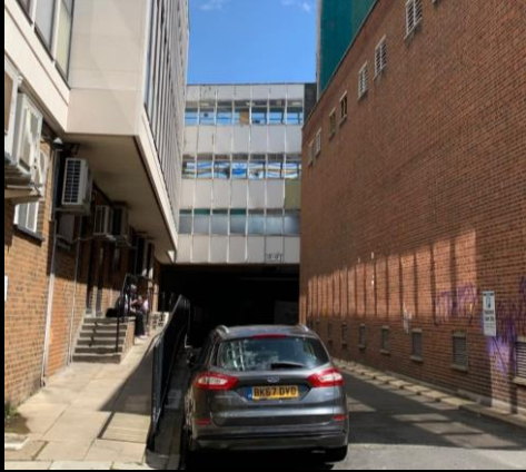
Existing Site Condition
